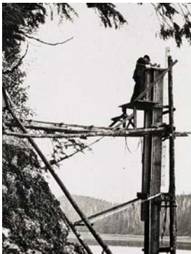
Figure 2. Automatic tide gauge at Port Protection, Prince of Wales Island, Alaska, 1915. Image credit: NOAA Photo Library.
